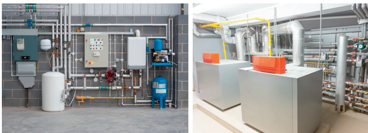
Figure 6. Examples of modern gas-fired boilers
