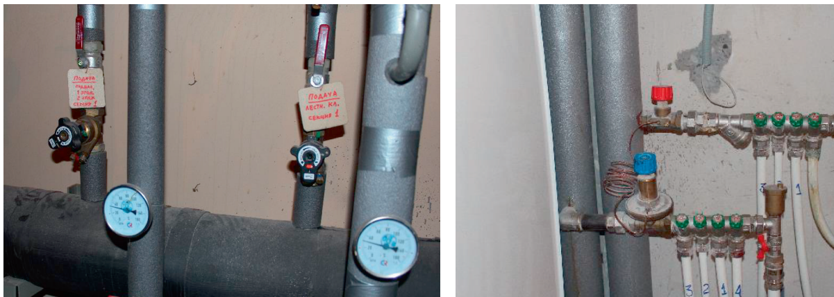
Figure 11. Example of balancing valves
