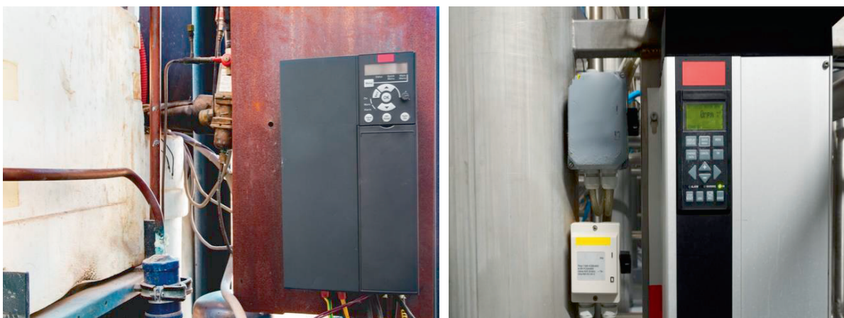
Figure 12. Frequency converters
