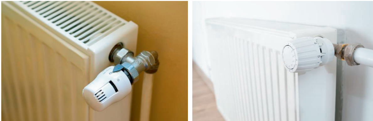
Figure 10. Thermostatic radiator control elements
