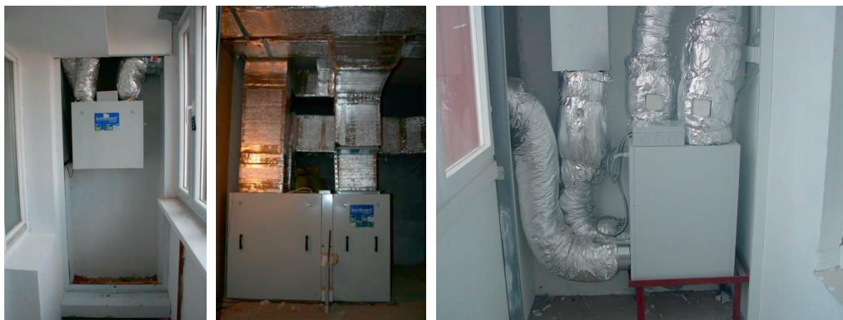
Figure 13. Heat recovery unit for mechanical inlet and outlet ventilation
