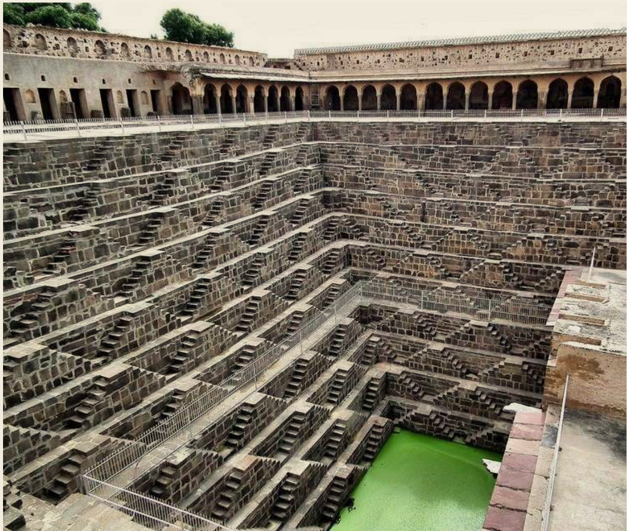
FIGURE 4.19 VIEW OF THE STEPWELL (SOURCE: KAUSHIK 2012)
